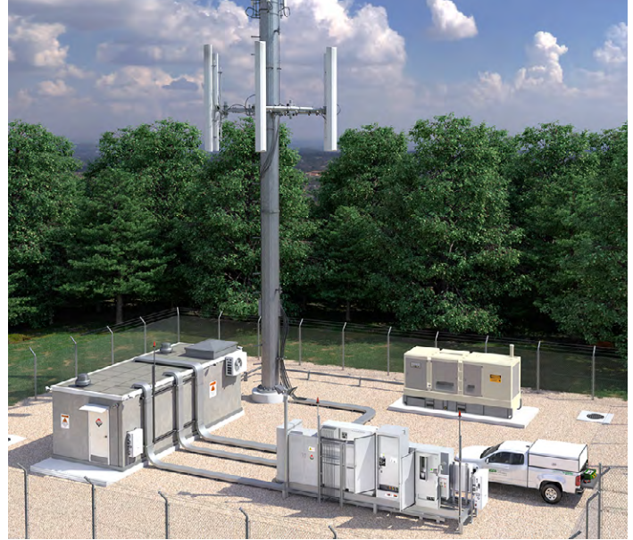
Providing a supplemental generator when a facility's sole permanent generator is offline
